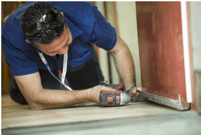
Figure SP6 Installation of under-door draught stopper
