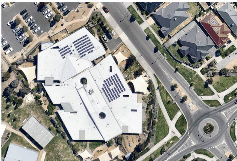
Figure SL7 Craigieburn Child and Family Centre solar panels
