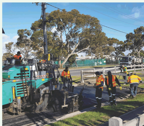
Figure SP1: Construction of recycled content road in Craigieburn
