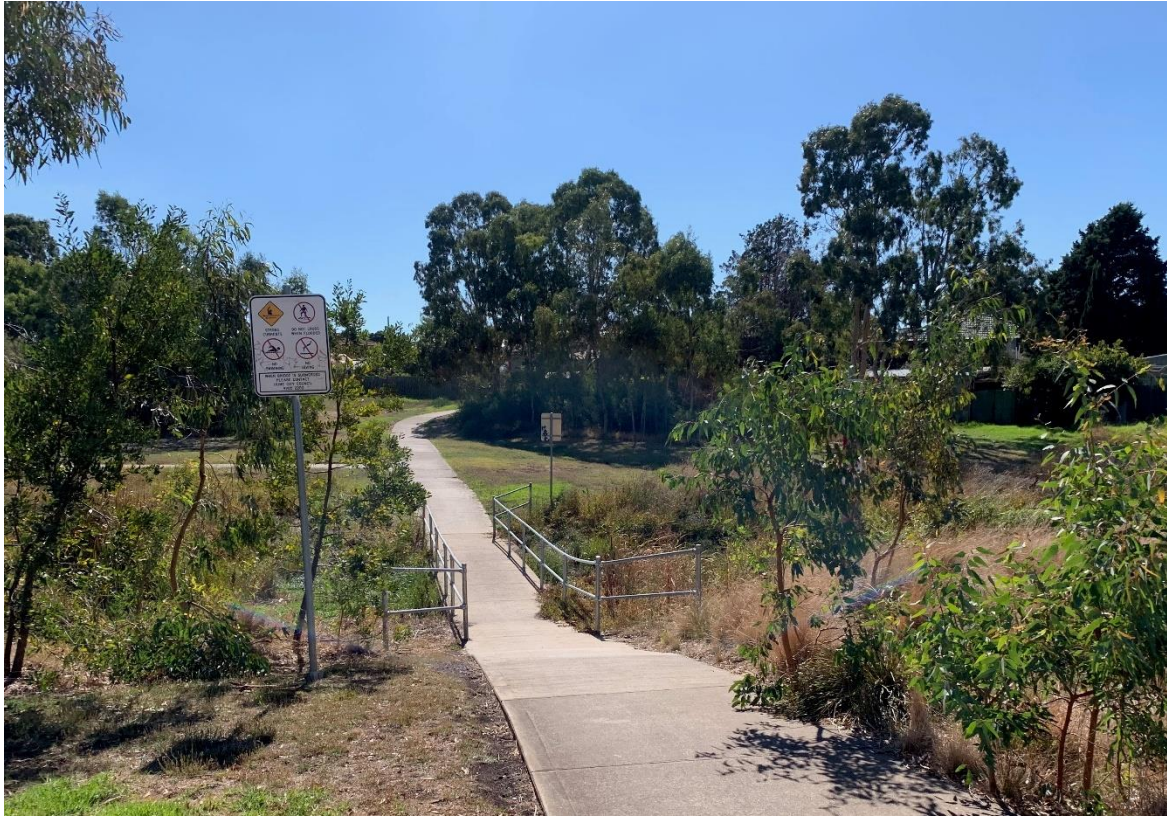
Existing low-level crossing – Axminster Drive side
