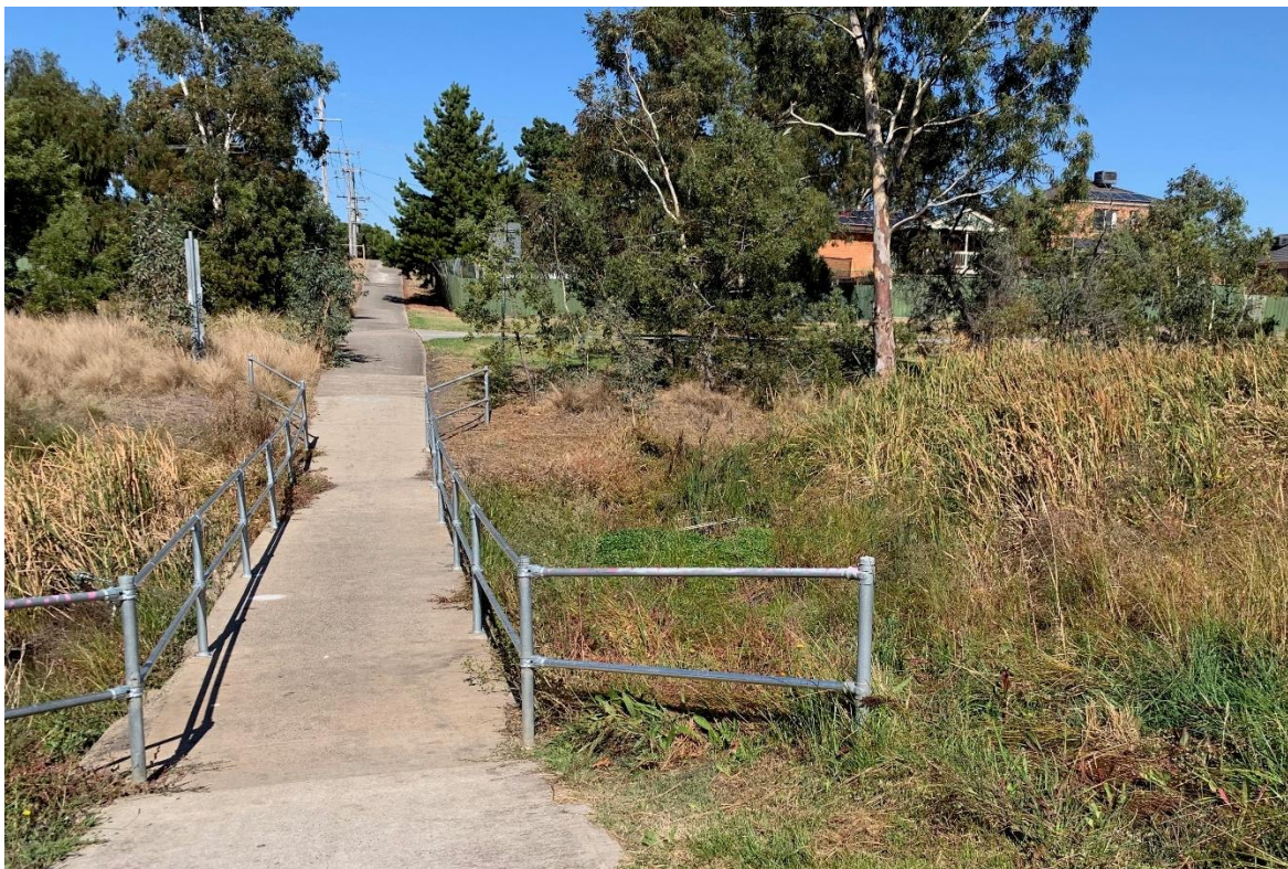
Existing low-level crossing – Clovelly Drive side
