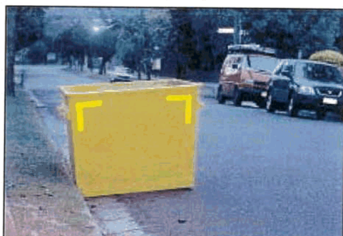
The waste bin should be placed so that vehicle access is not affected.
