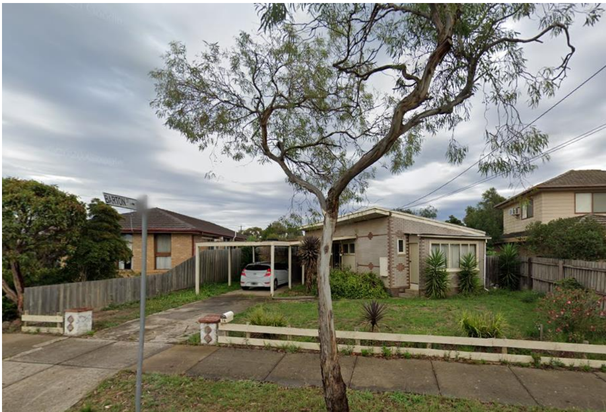
Figure 3 - Subject site – existing presentation to the street – 14 Flinders Street, Sunbury (Google Maps, 2022)
