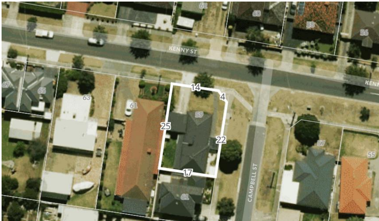
Figure 6 - Aerial of southern interface (Landchecker, 2020)
