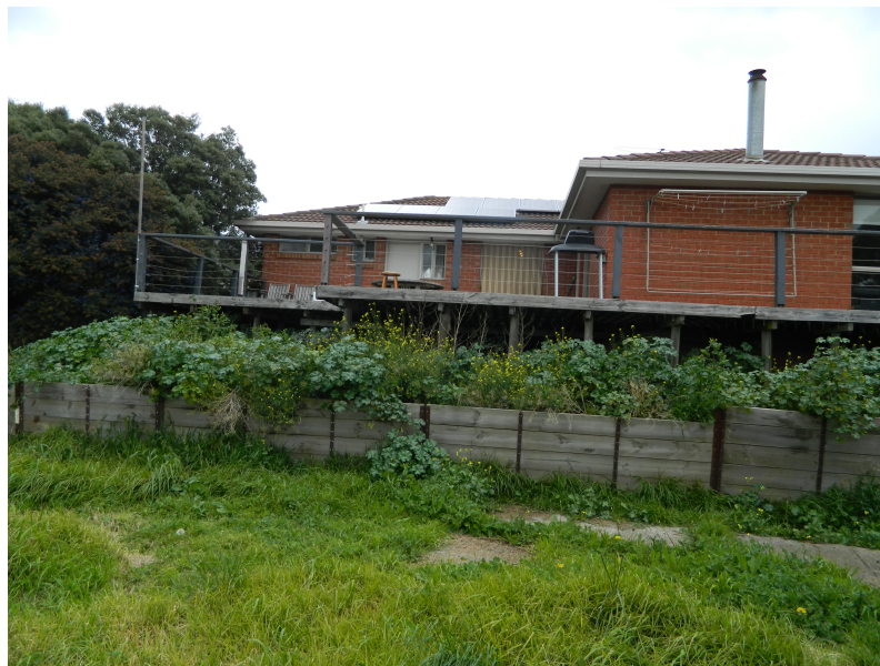
looking to South at existing Dwelling
