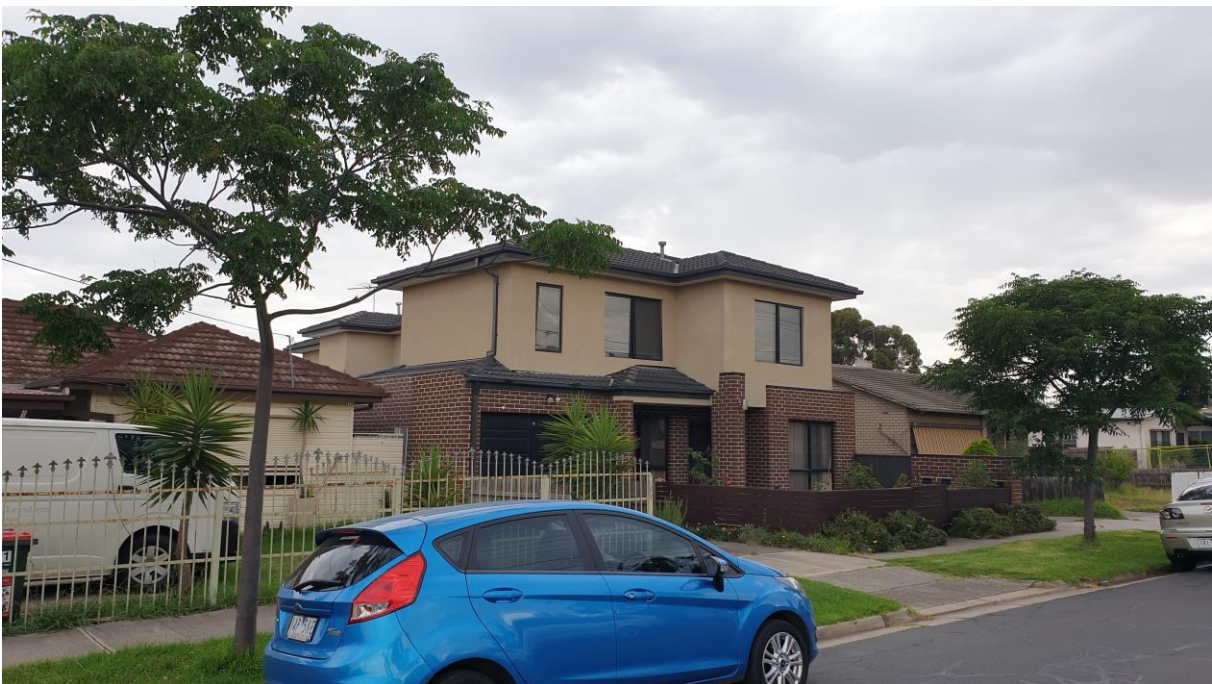
Figure 10 Eastern neighbour, abutting, 43 Cuthbert Street, north east elevation.
