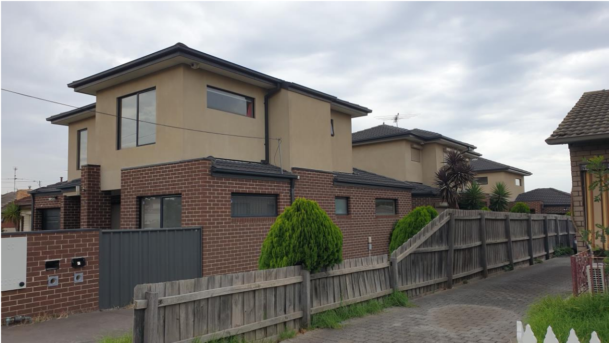
Figure 9 Eastern neighbour, abutting, 43 Cuthbert Street, north west elevation.
