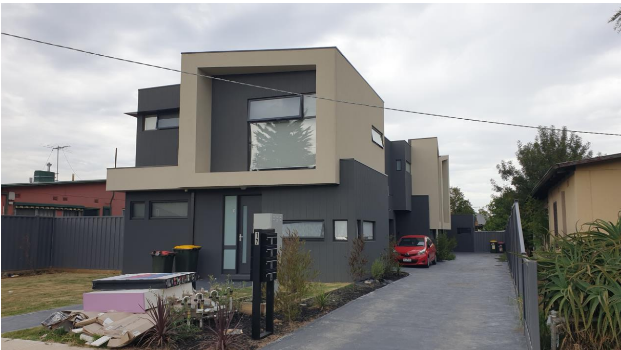
Figure 12 Local infill development at 17 Cuthbert Street, continuous built form across the length of site
