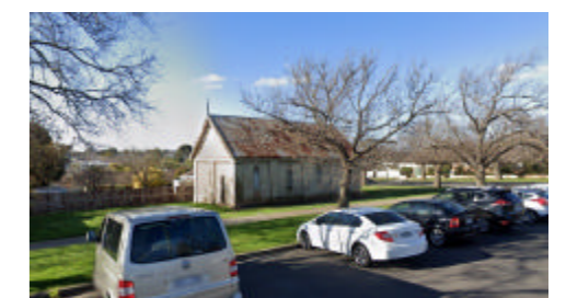
ADJOINING PROPERTY - No. 23
