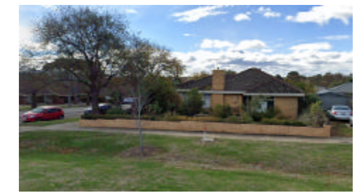
ADJOINING PROPERTY - No. 25
