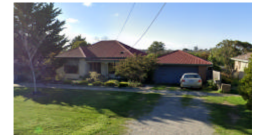
ADJOINING PROPERTY - No. 15
