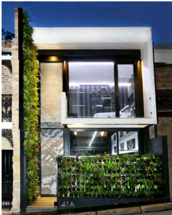
VERTICAL GREEN WALL
