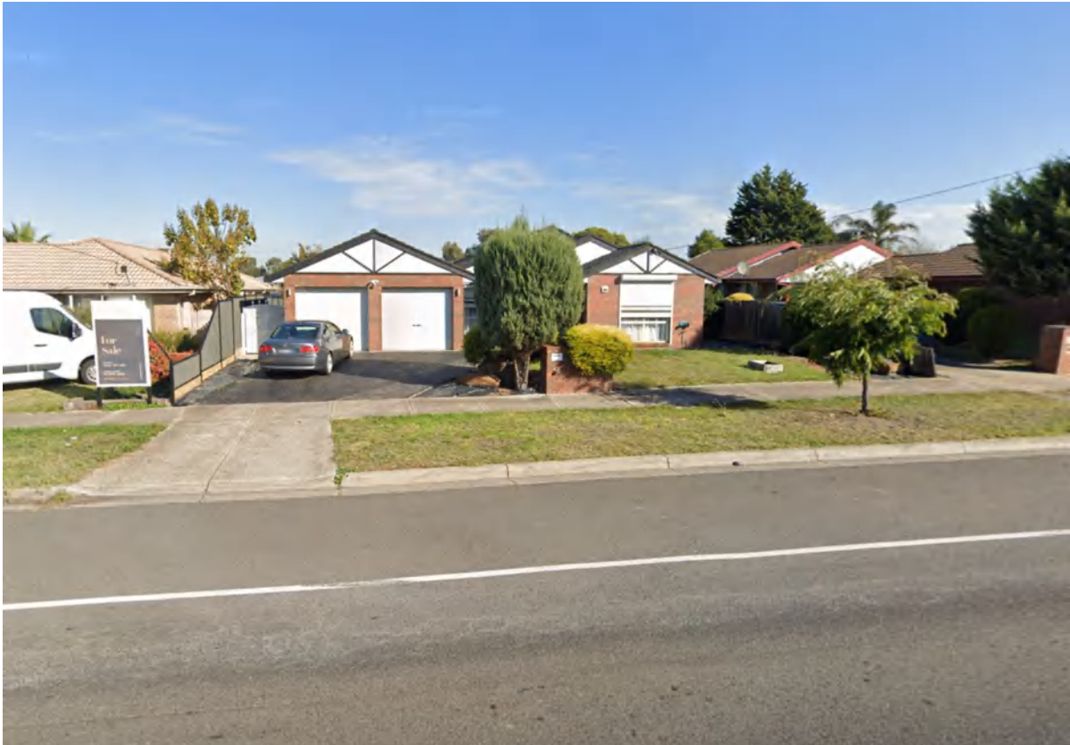
Figure 4: Views onto the adjoining dwelling to the west
