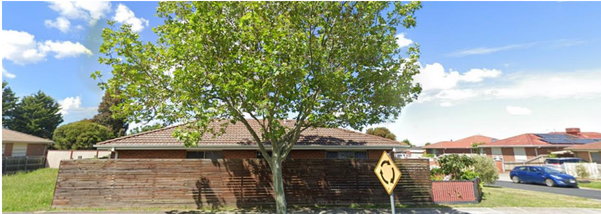
Figure 4: Left-side view of the proposed site from the Paringa Boulevard
