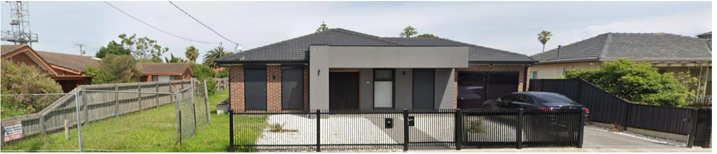
Figure 1: Subject Site (3 Joffre Street, Broadmeadows interface)
