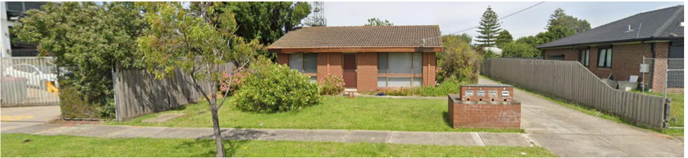
Figure 3: Subject Site (1/1 Joffre Street, Broadmeadows interface)
