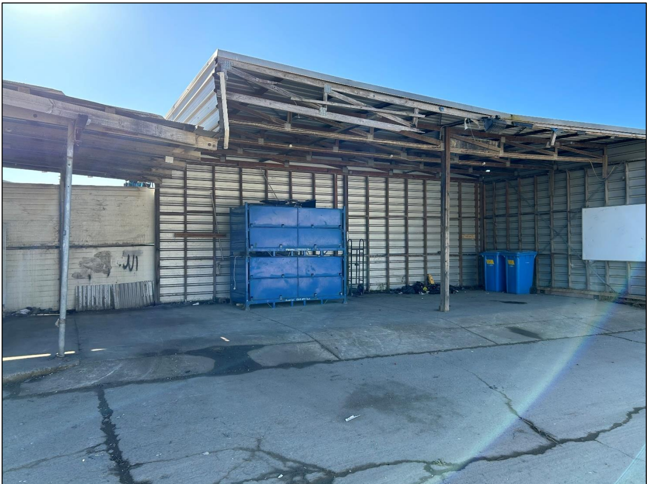
Figure 6-1 E-Waste Storage Shed
