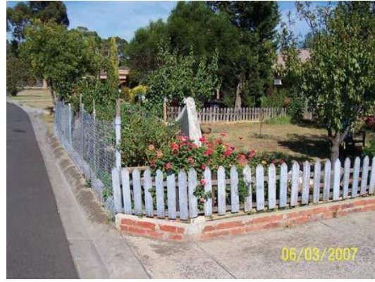
Pedestrian access blocked and tripping hazard.
